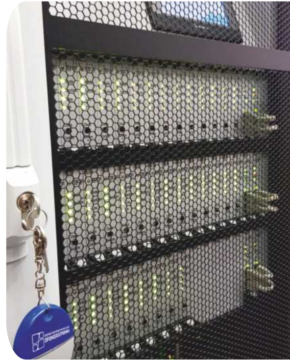
ESSO-M-2 indoor equipment
