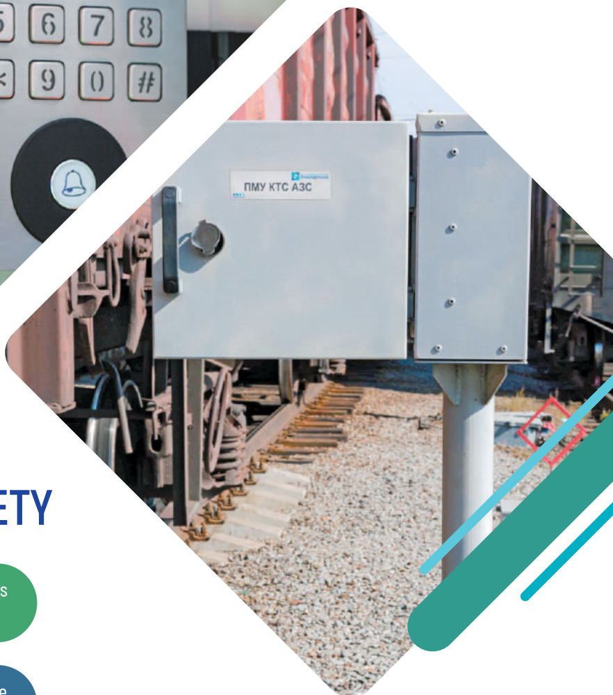
Local control panel
