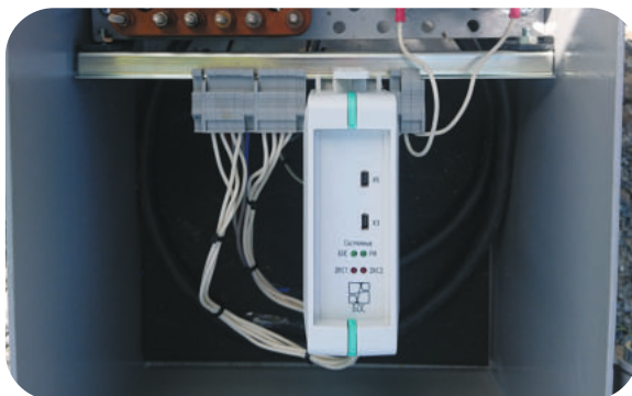
BOS Signal Processing Unit
