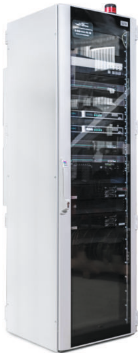
ShTK Communications Cabinet
