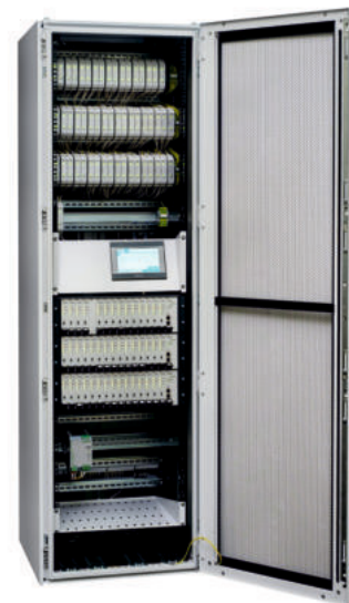
ESSO-M tower equipment
