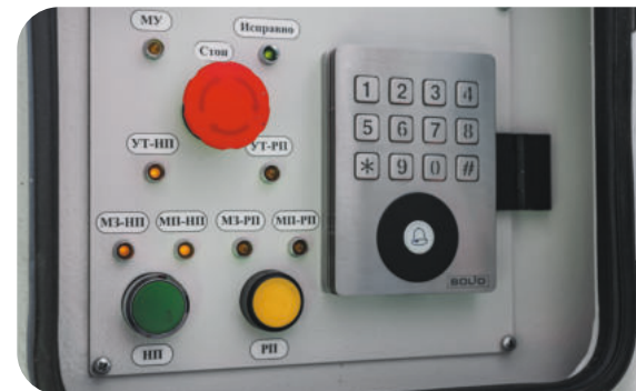
Local Control Panel
